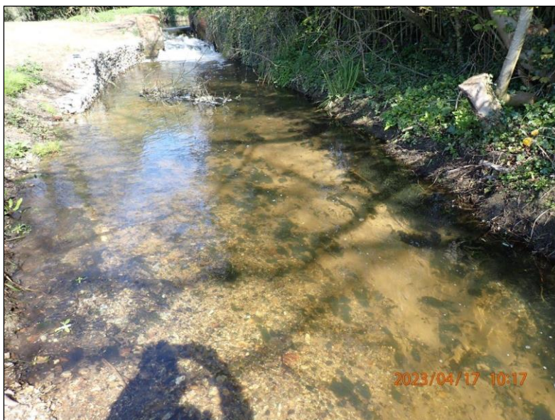
Photograph 8. (Exhibit AM01H-P4170003) Bypass channel showing reprofiled banks and disturbance to gravel bed.
