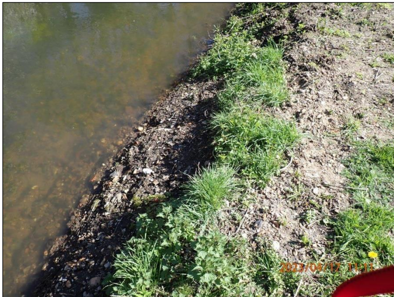
Photograph 2. (Exhibit AM01B-P4170024) Reprofiled bank edge and gravel deposited on bank top. Upstream end of reach.
